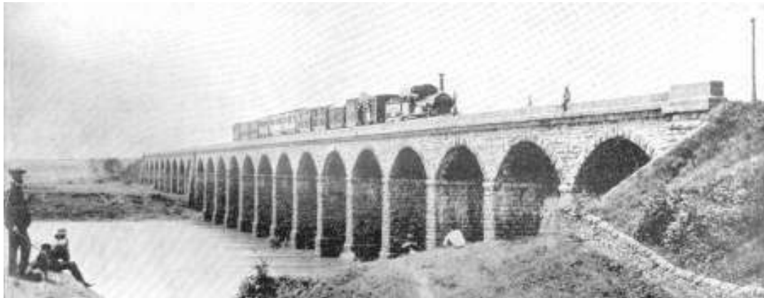
Fig. 1.4 First Railway Bridge linking Bombay with Thane, 1854
